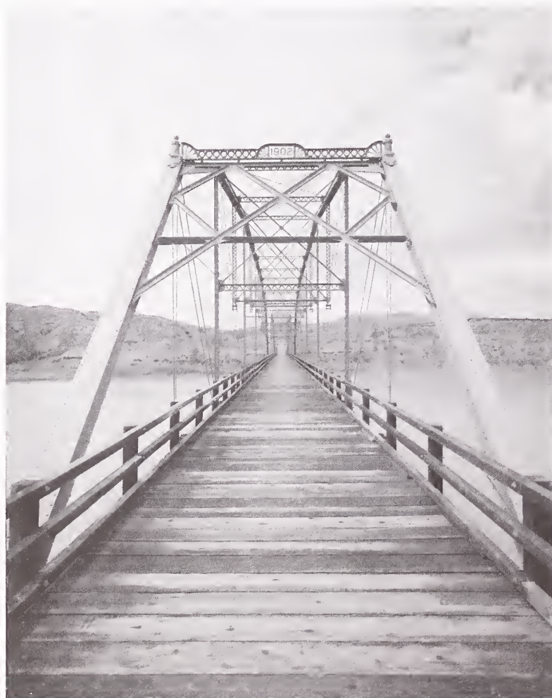
The Fort Keogh Bridge. (HAER Photograph by Jet Lowe).
